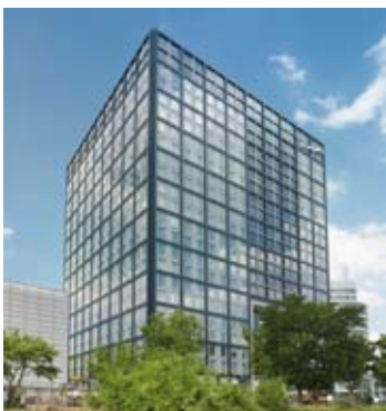
TRANSPARENT, EFFICIENT, ENVIRONMENTALLY-FRIENDLY: THE NEW EXCHANGE HEADQUARTERS.
